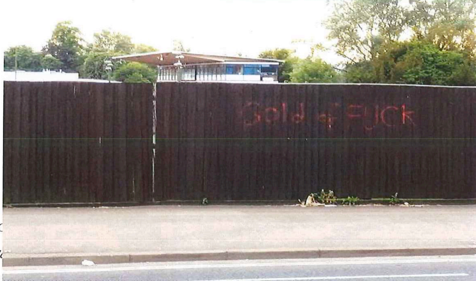
2 places along Perimeter Fence of Oxford Sports Centre, Iffley Road
